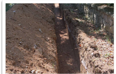
Excavations of the sewer network
