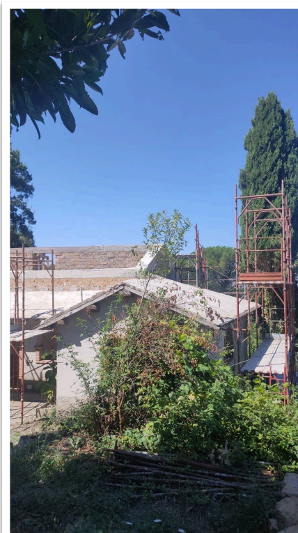
Retaining of the roofs
