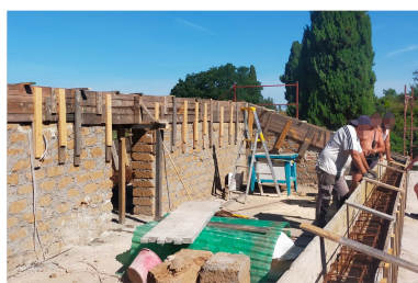
Demolitions, deforestation and external reorganization to the guesthouse
