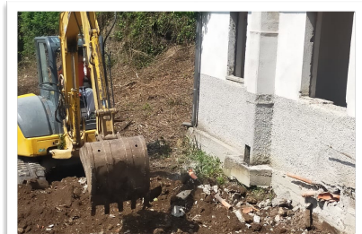
Demolitions, deforestation and external reorganization to the guesthouse
